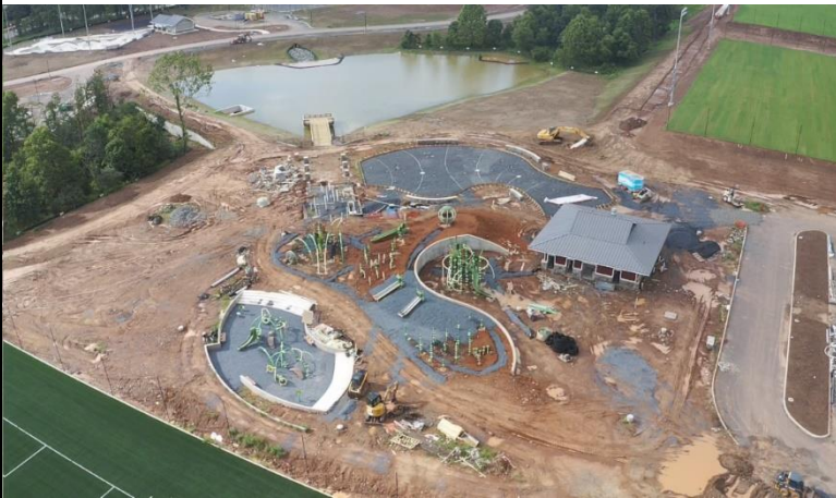
Construction progress on the playground
