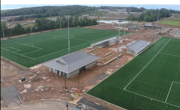
Construction progress on the athletic fields
