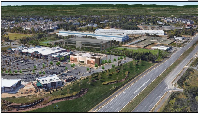
View looking west along Route 50
