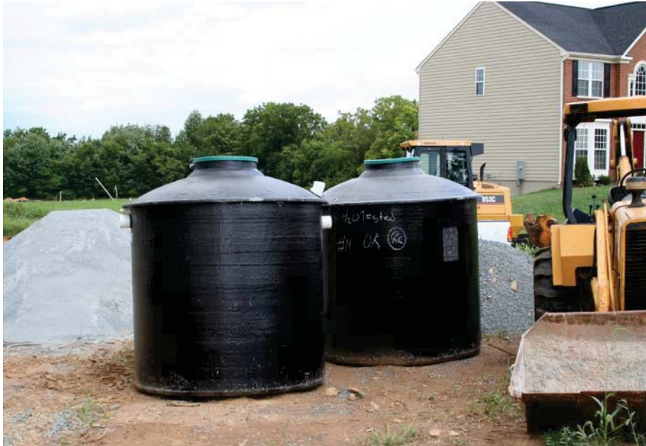
Two Aerobic Treatment Units (ATU's) awaiting installation
