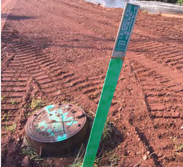
Figure 8. Sanitary Line Along Lockridge Road West and Prentice Drive
