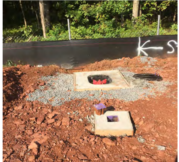
Figure 10. Installation of a New Water Valve
