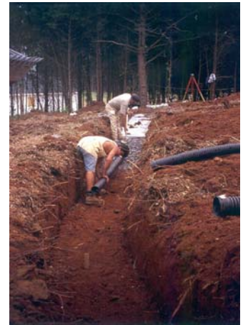
Gravel Trench Under Construction
